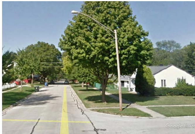
ComEd owned street light located at the intersection of Elm Street with Isabella Street.
