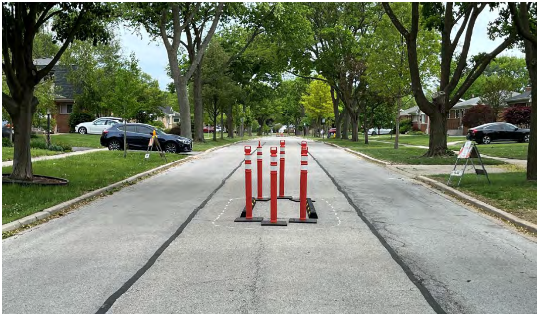
Example Temporary Median Island Installed on Hatlen Avenue
