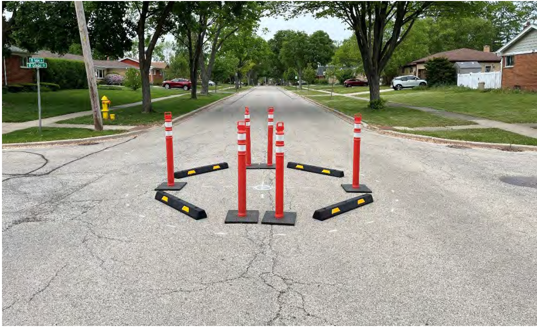
Example Temporary Mini Traffic Circle Installed on Hatlen Avenue at Grindel Drive
