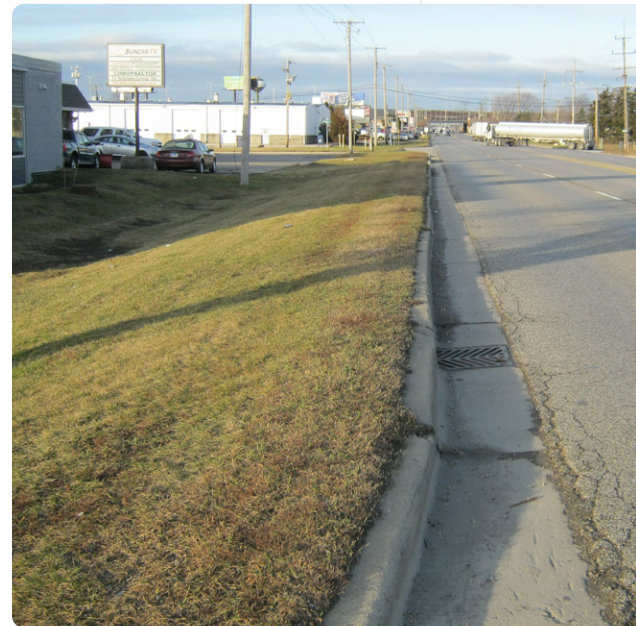
Right: Sidewalk gap along a Pace bus route on Oakton Street (looking west on south side of Oakton at Elizabeth)
