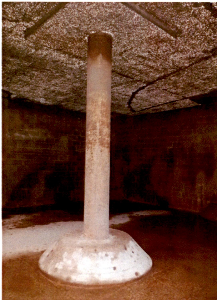
26. Column and tank interior.
