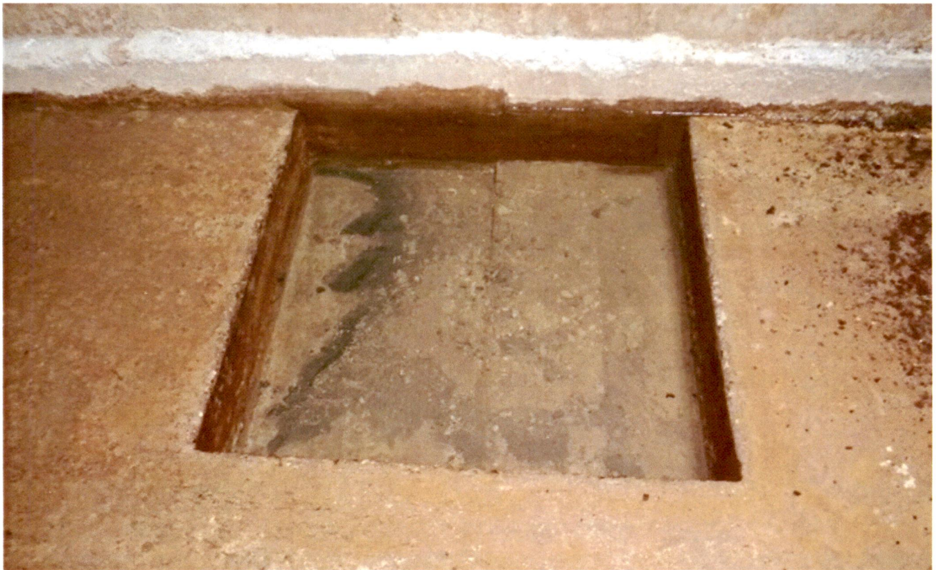
54. Sump in floor.
