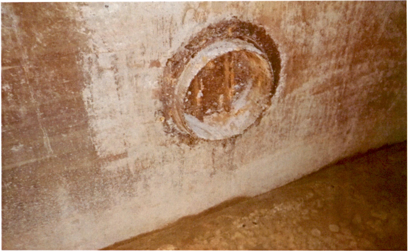
47. Sealed opening in shell.
