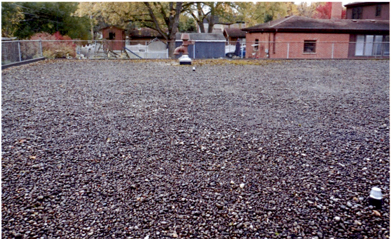
8. Tank roof and roof vent.
