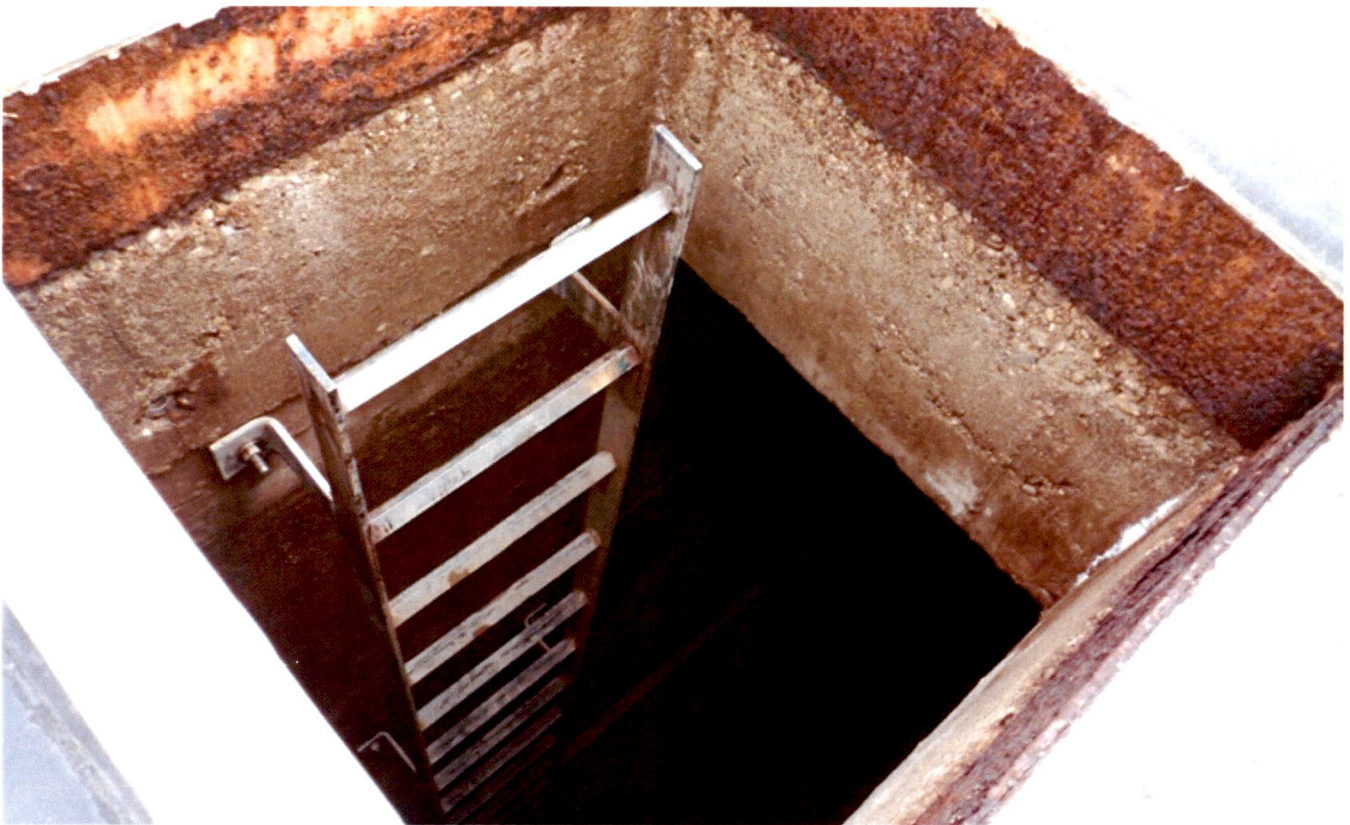
20. Roof manhole and interior ladder.
