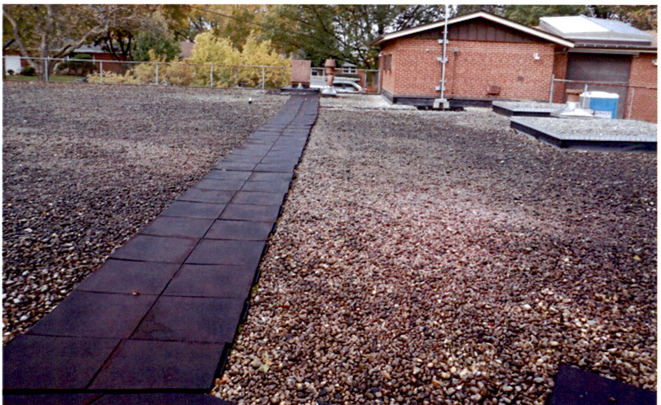
4. Tank roof and walkway between roof manholes.
