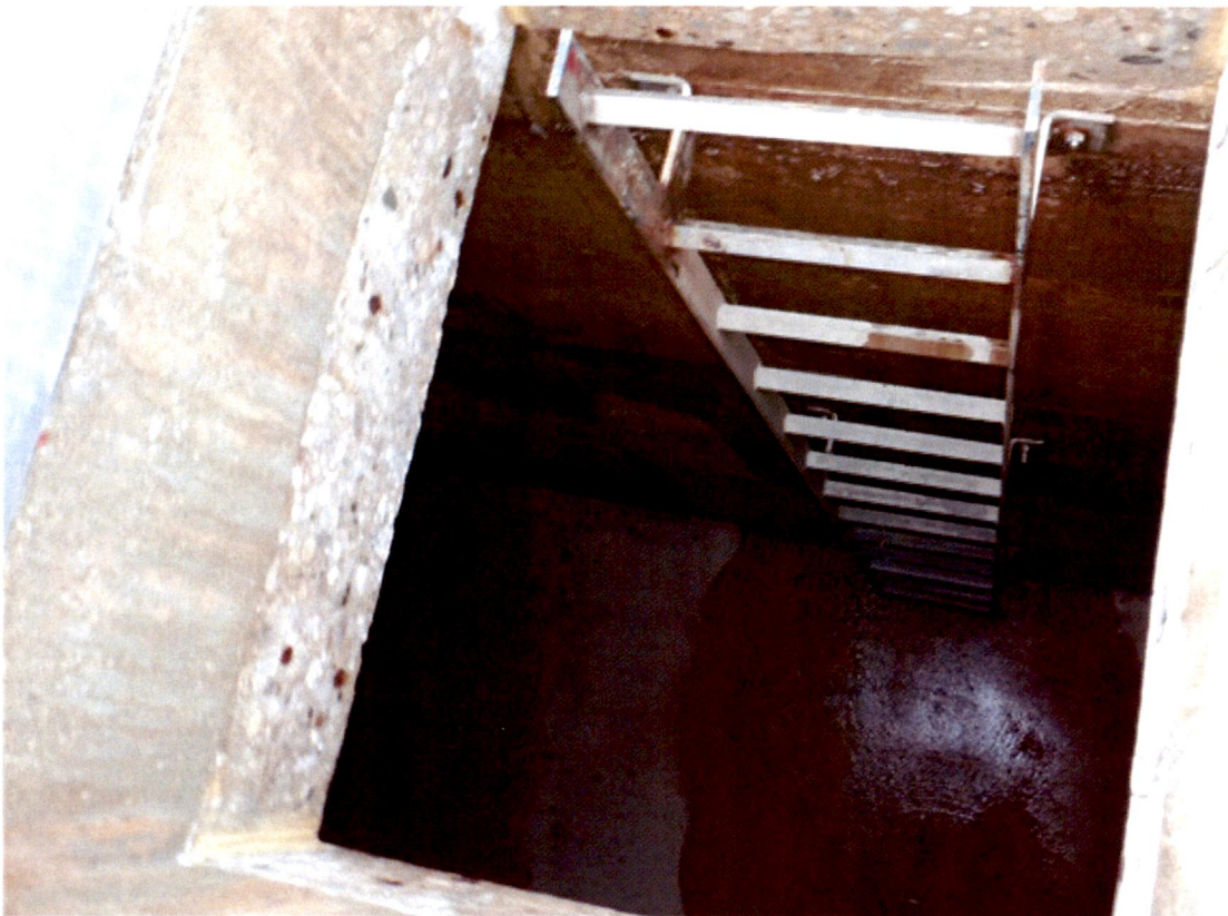
22. Roof manhole and interior ladder.
