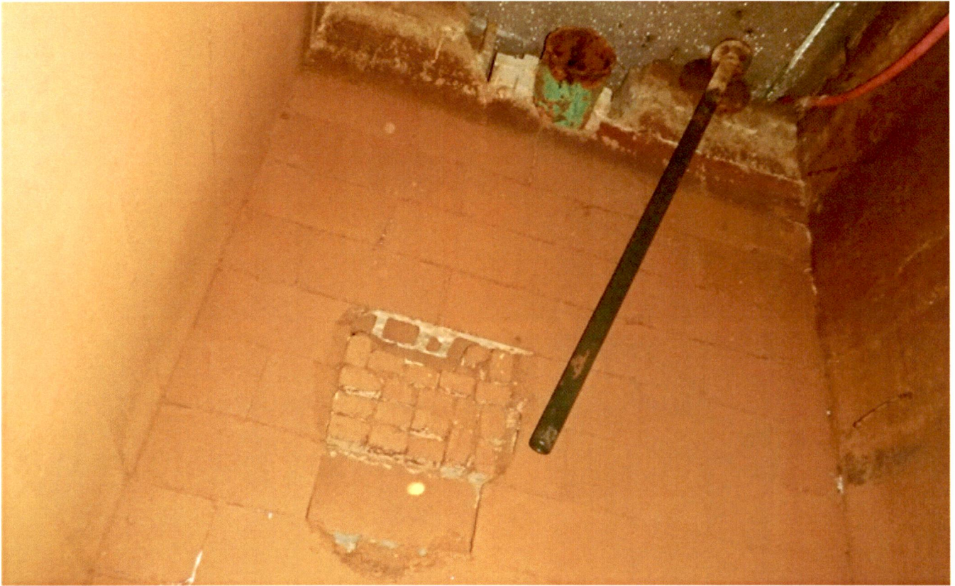
39. Pipe penetrations in roof.
