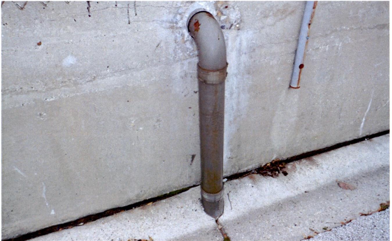
7. Pipe that penetrates shell wall.
