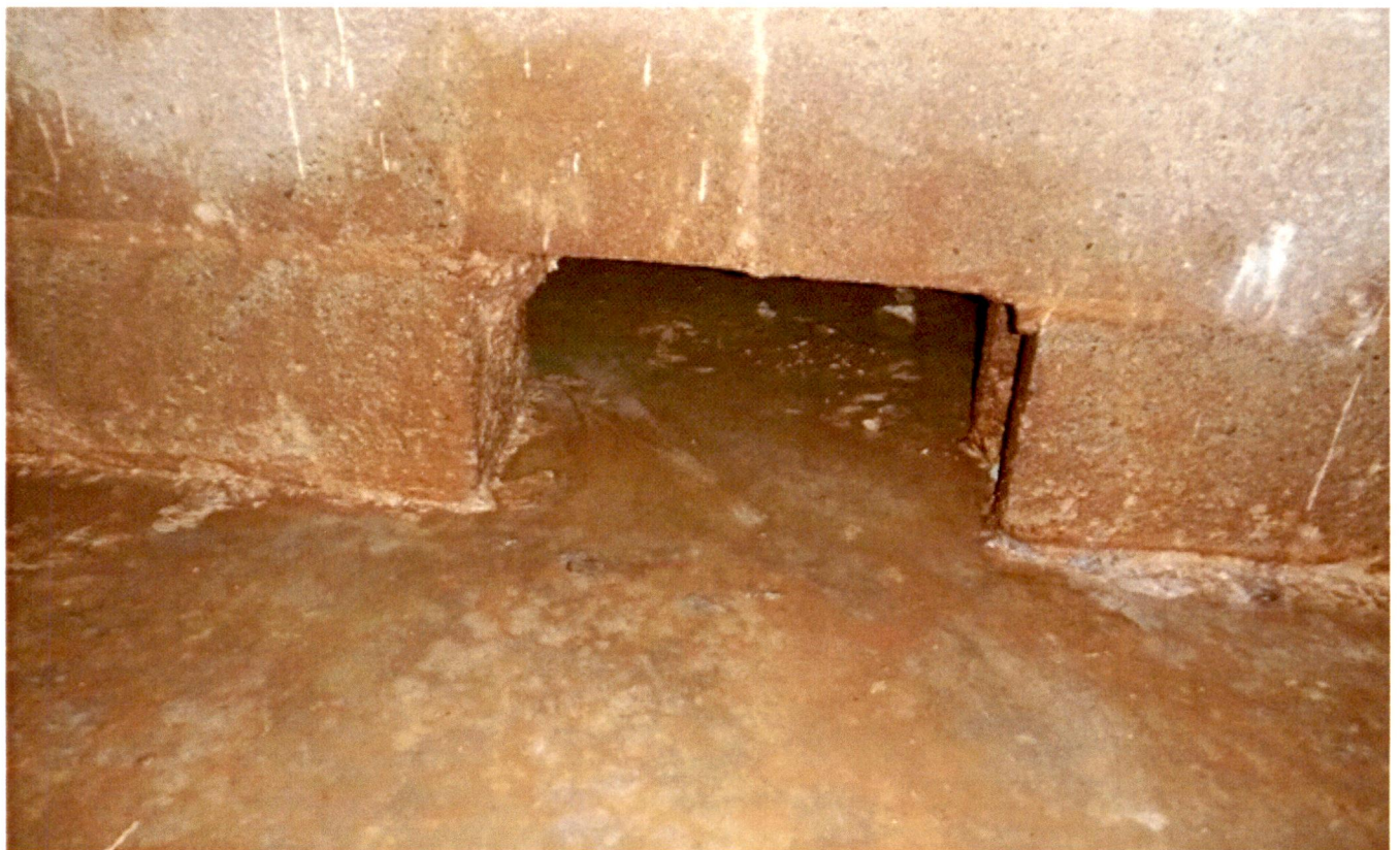
46. Opening at base of baffle wall.
