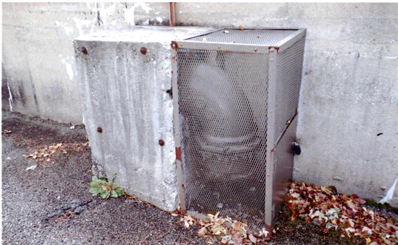
6. Overflow pipe and enclosure.
