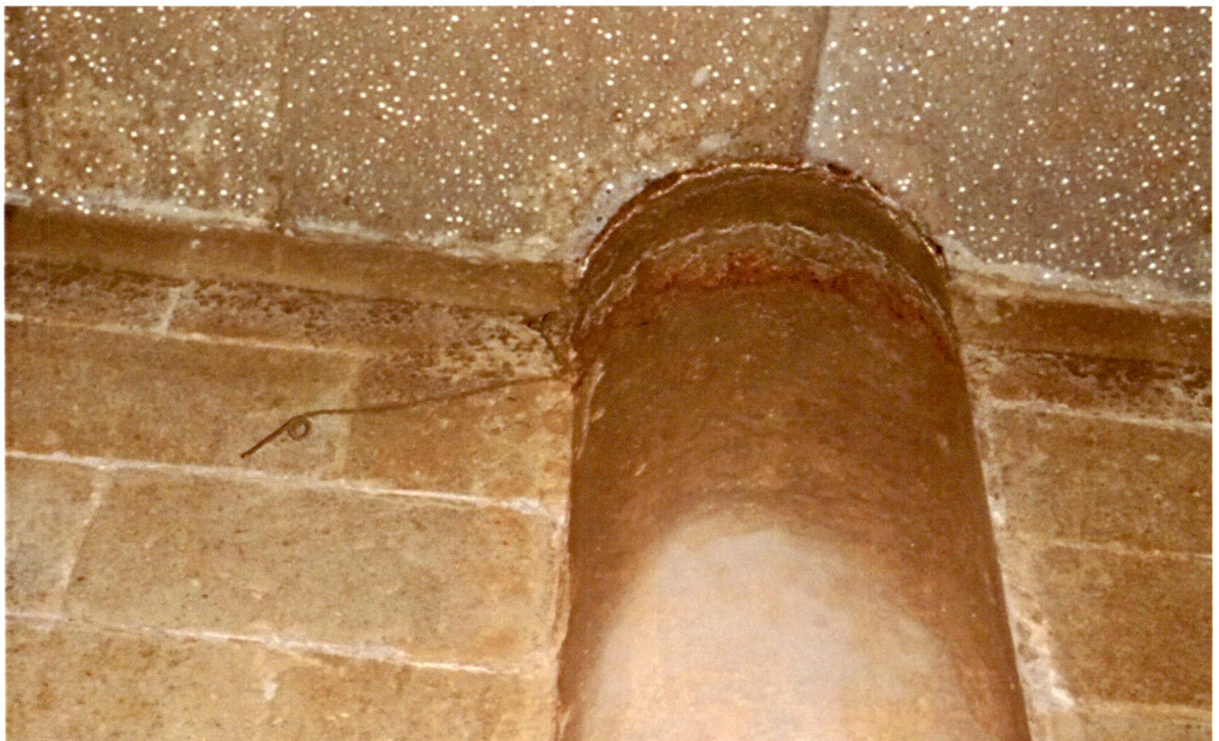
34. Baffle wall, column, and roof.
