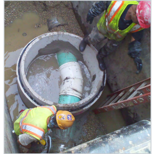
We have a long history helping the Village reduce I/I and proactively maintain your sewer system infrastructure! The photo above shows spot repairs being constructed on Route 83 during your 2011 rehabilitation program.
