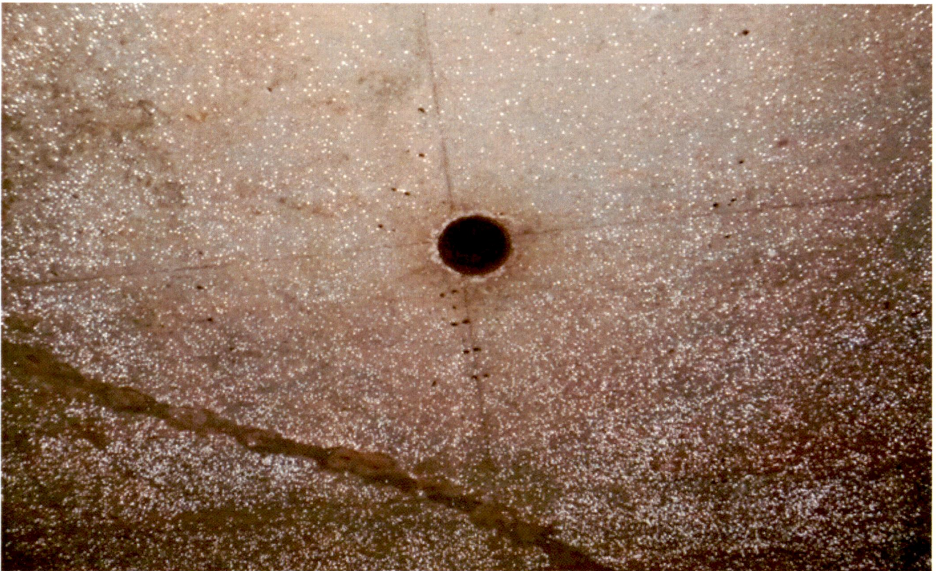
32. Opening in tank roof.
