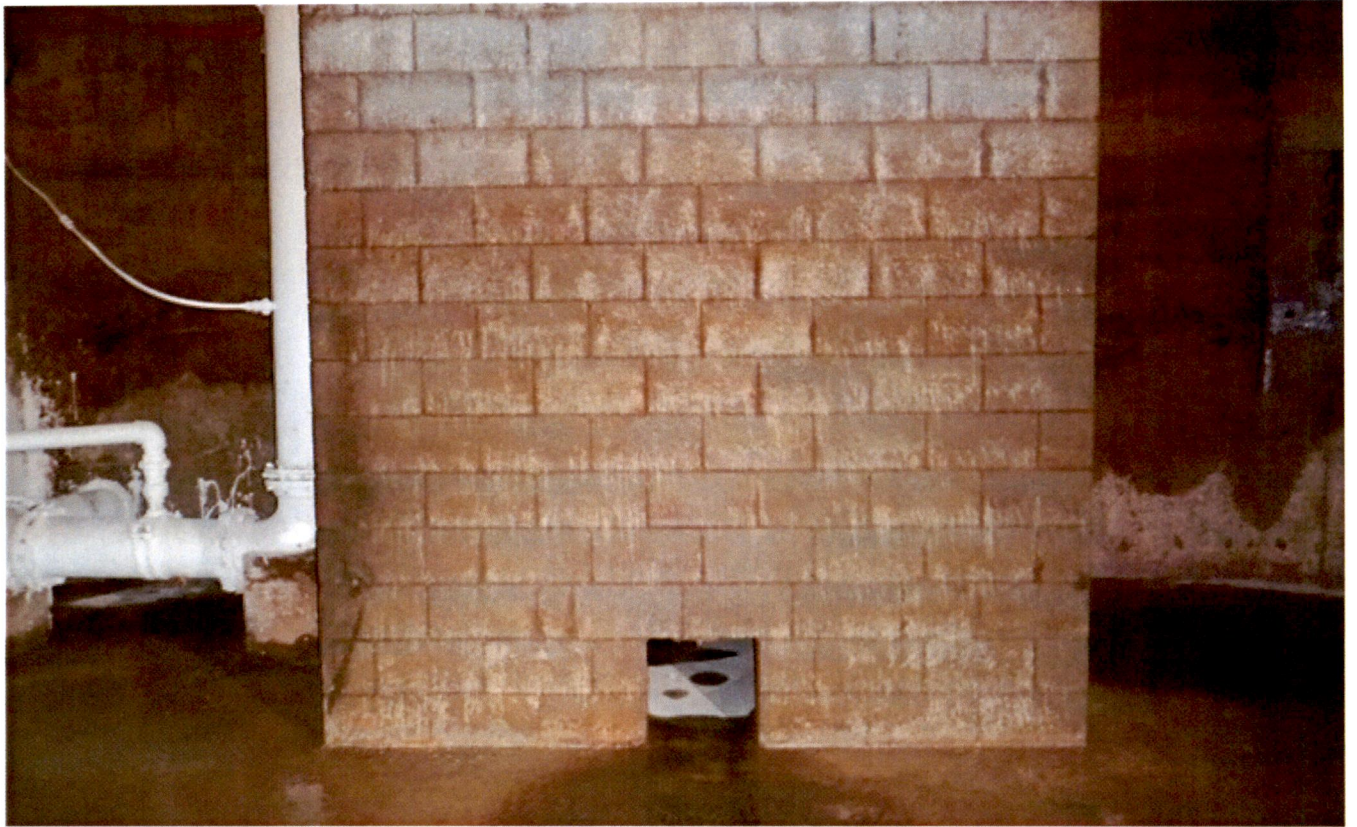
43. Opening at base of baffle wall.
