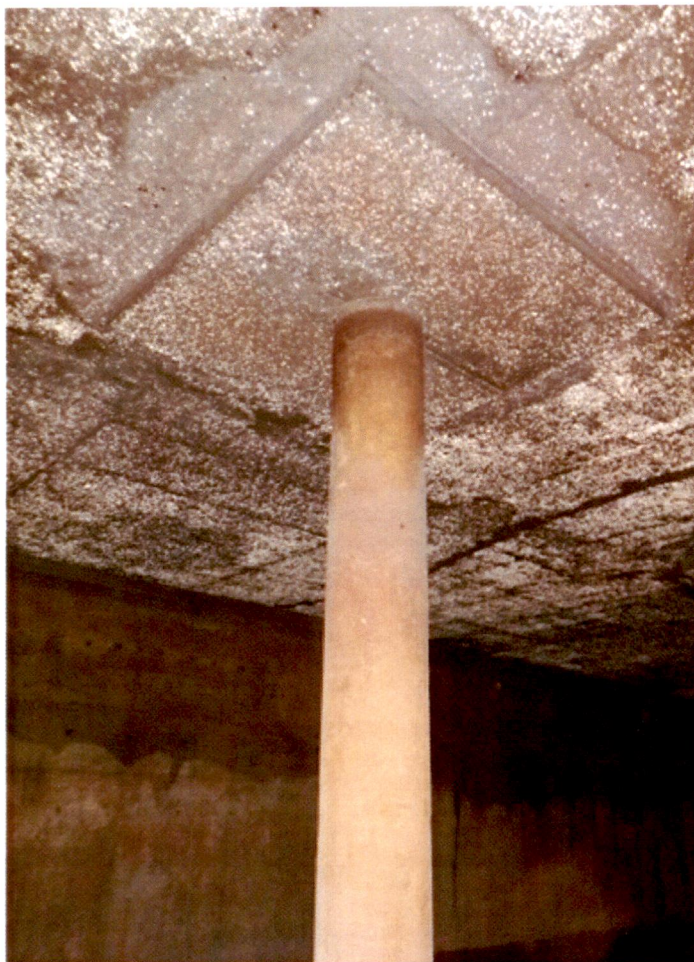
25. Column and roof interior.
