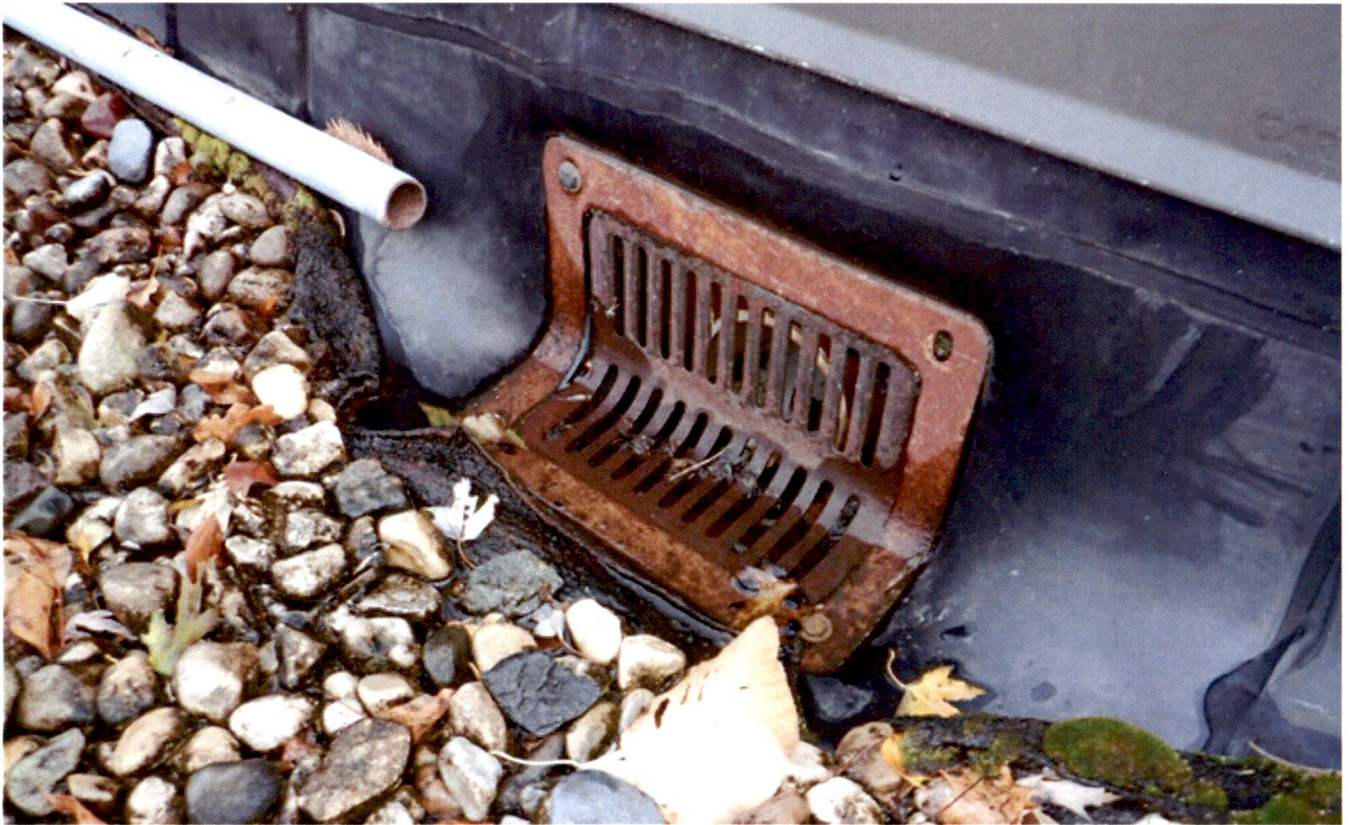
11. Grate-covered drain in tank membrane.
