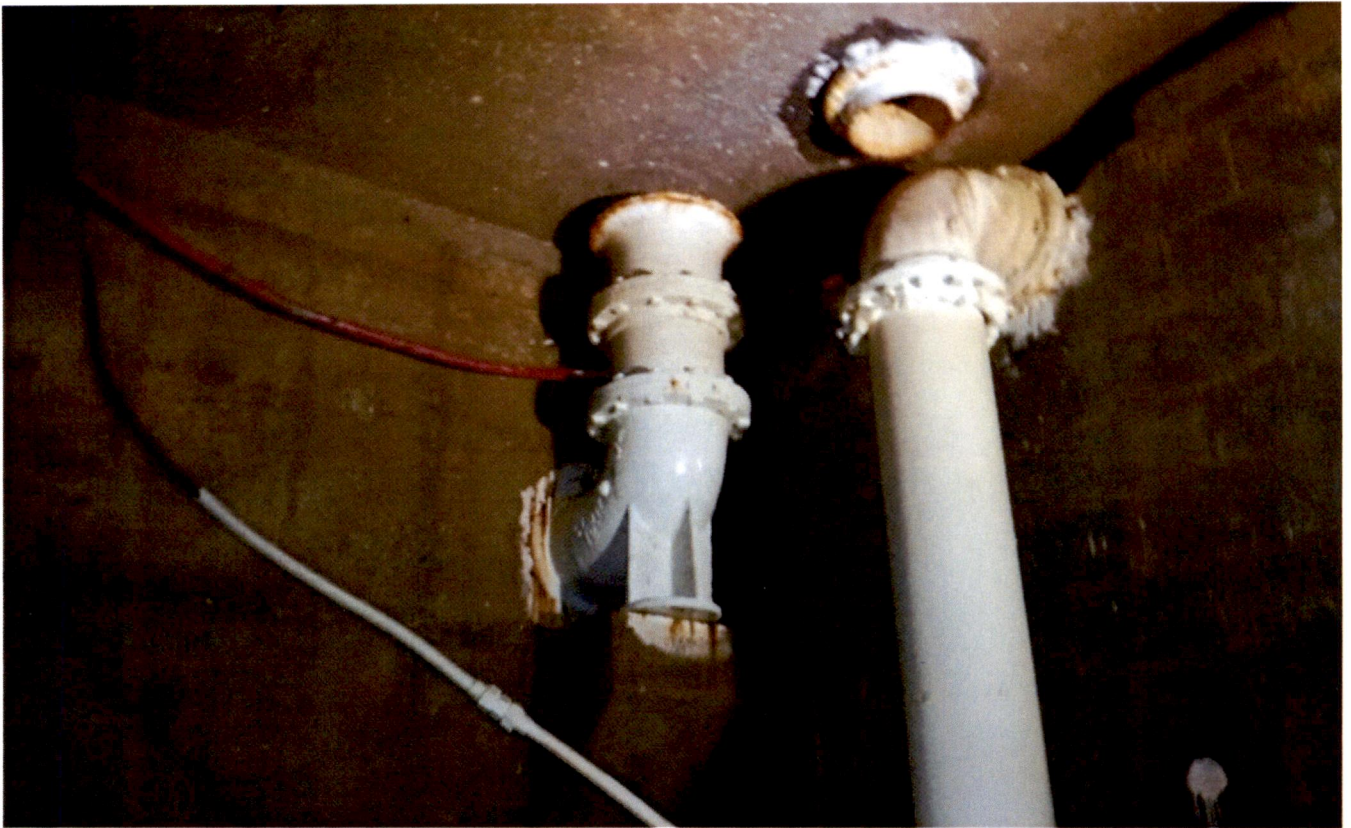
57. Overflow inlet, pipe penetration in roof, and interior piping.
