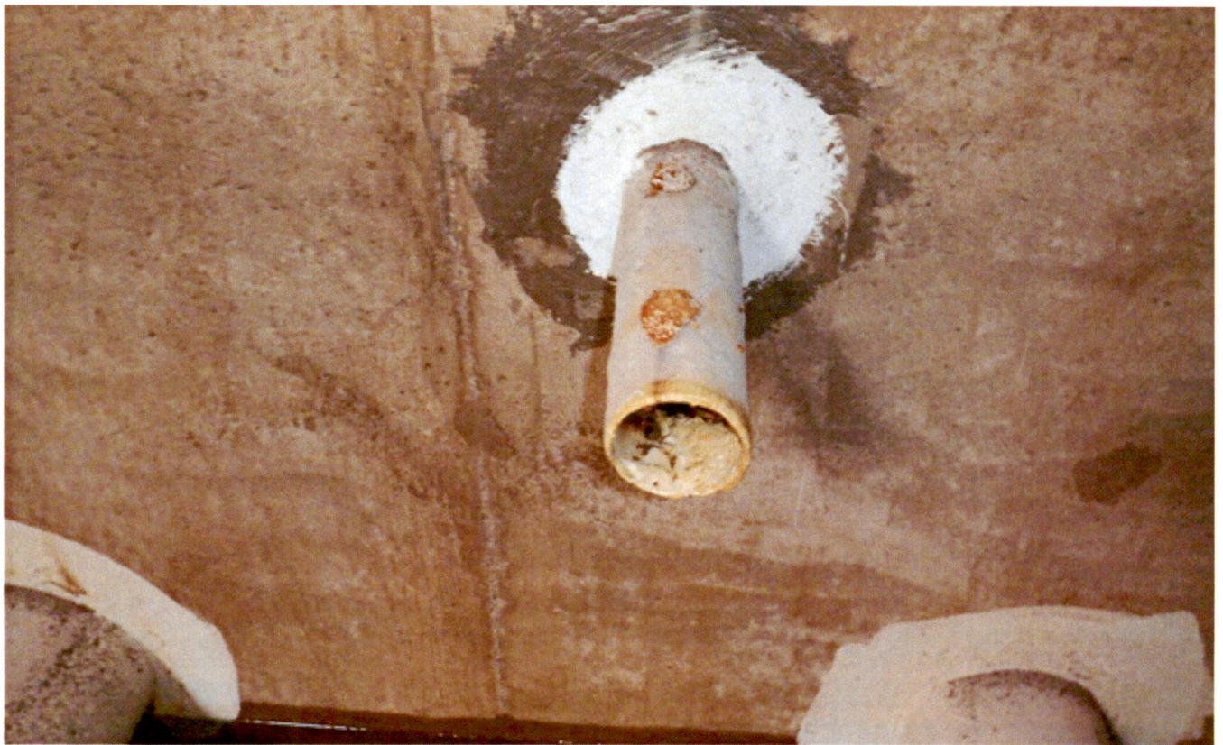
56. Pipe penetration in roof.
