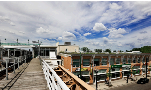
Bethel Commercial Center Transit-Oriented Development | Chicago, IL
