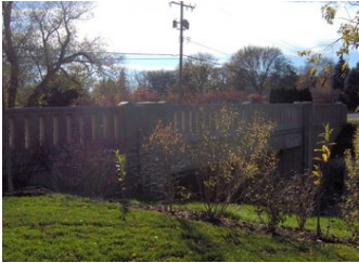
Lincoln Street Bridge
