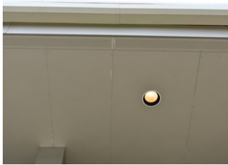
Fire Station 14 Exterior Painting
