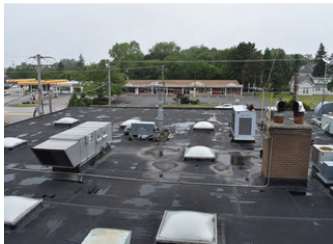
Fire Station 12 Roof Replacement
