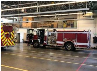
Fire Station apparatus floor wall painting
