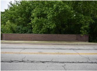
Business Center Drive Bridge
