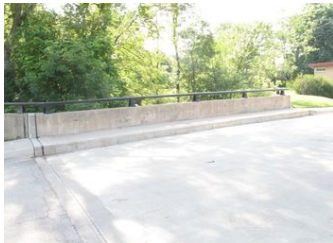
Seegwun Avenue Bridge
