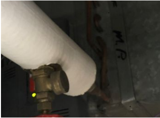
PW HVAC VAV box replacement
