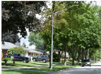
Residential Street Lighting
