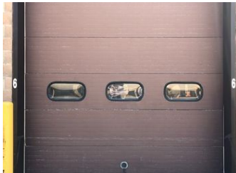
Public Works Overhead Door Replacement
