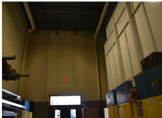
PW Vehicle Shop Painting
