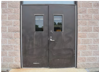
PW Exterior Door Replacement
