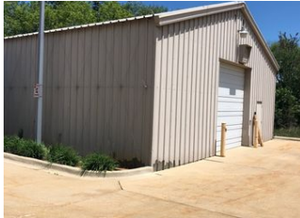
Fire Station 14 Butler Building Maintenance
