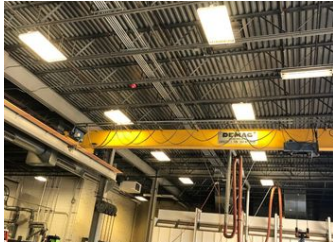
PW vehicle Maintenance lighting retrofit
