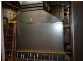
HVAC Replacement Program
