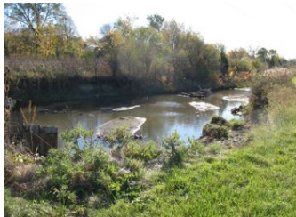
McDonald Creek Bank Stabilization
