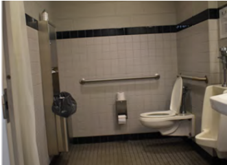
Fire Station 12 Bathroom Remodel
