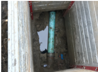
Sanitary Sewer Spot Repair
