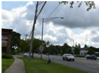
Street light pole
