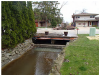
Briarwood Drive West - South Bridge
