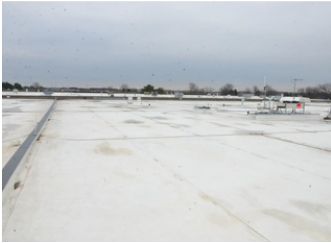
PD Roof Replacement
