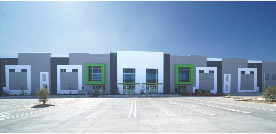
Figure A.6 An example of an extreme approach to breaking down scale that is being demanded in some cities.
