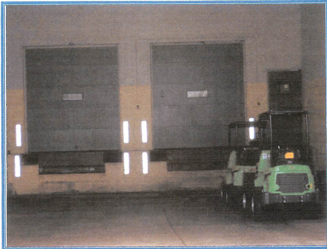
Front loading dock
