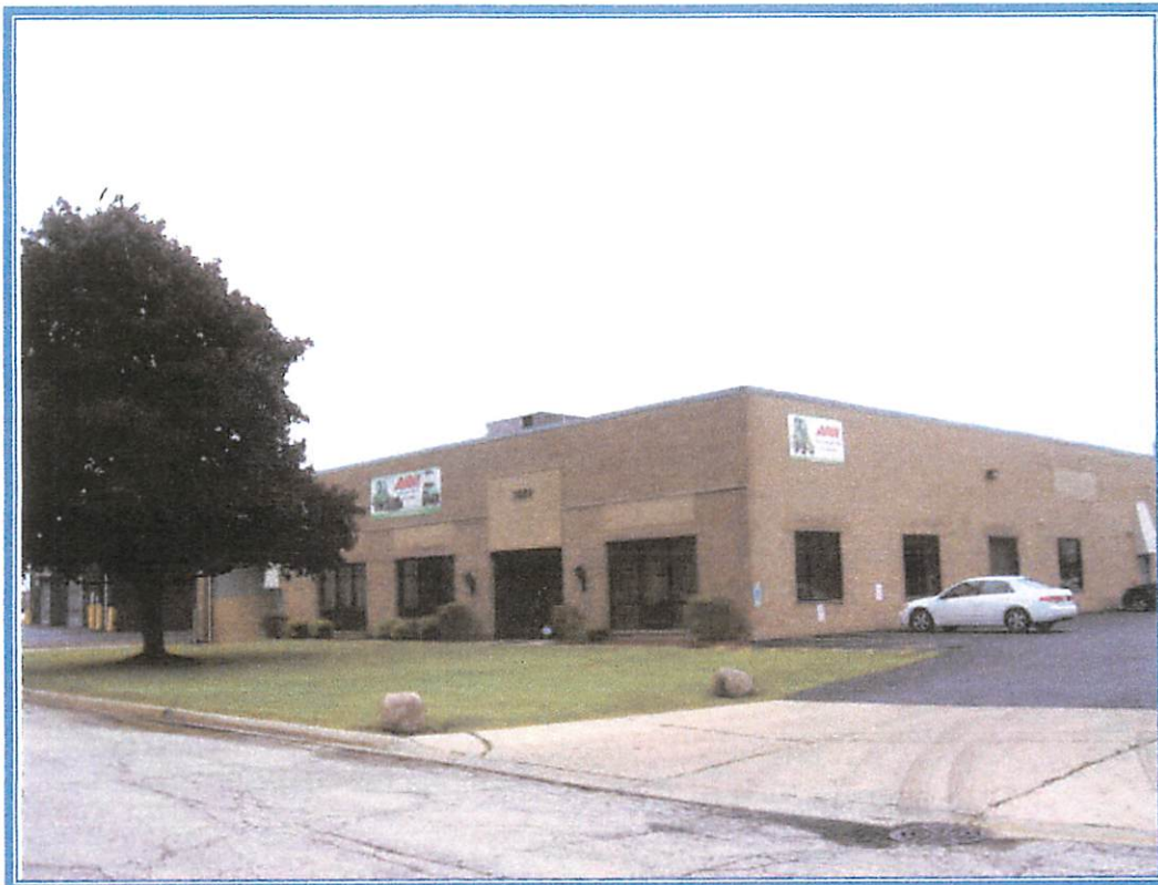
East (front) & north elevation – looking southeast
