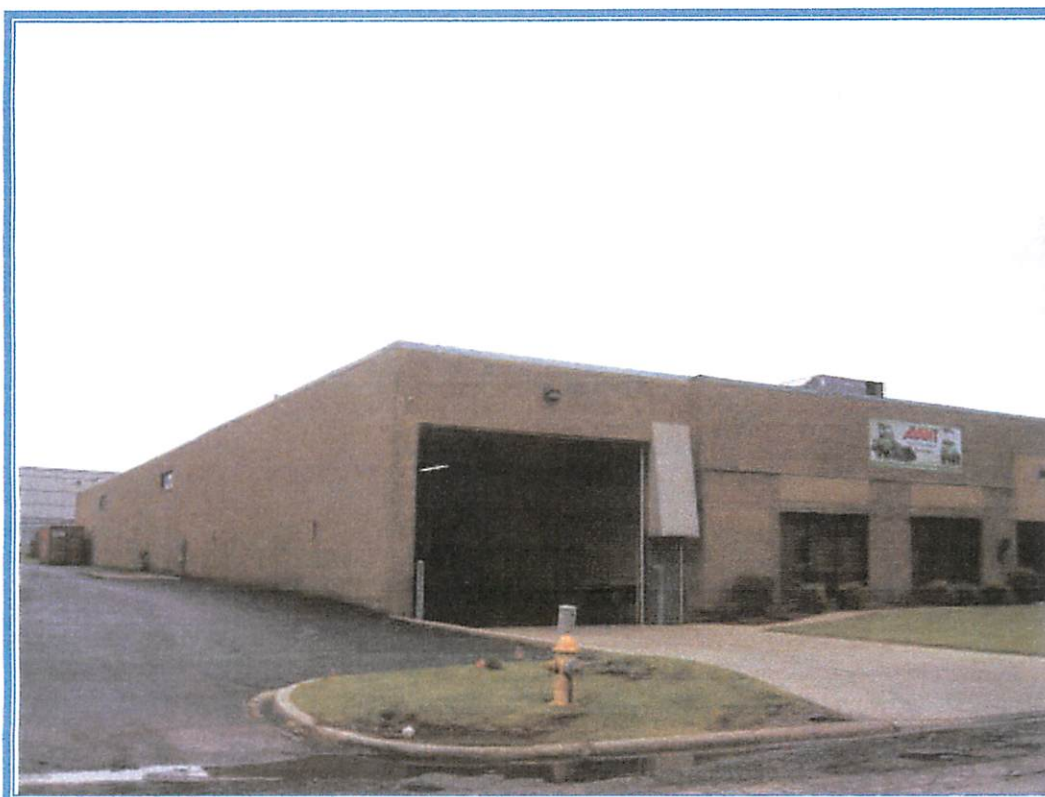
South and east elevations – looking northwest
