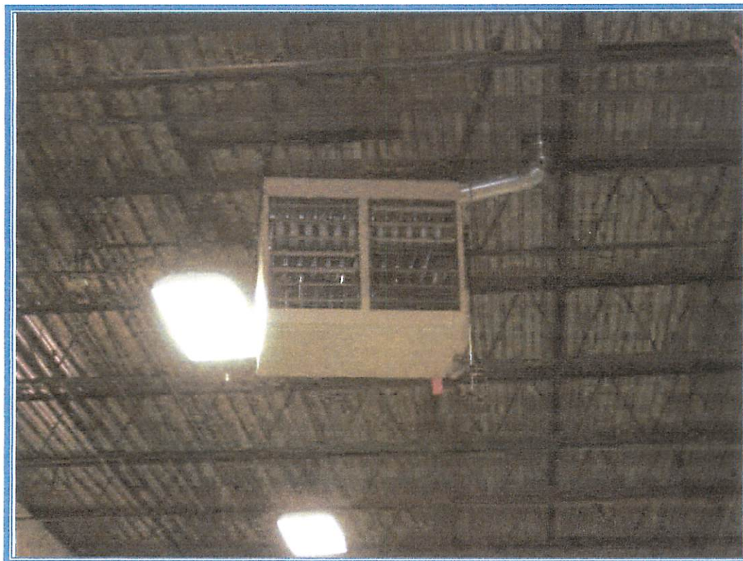
Ceiling hung heating unit
