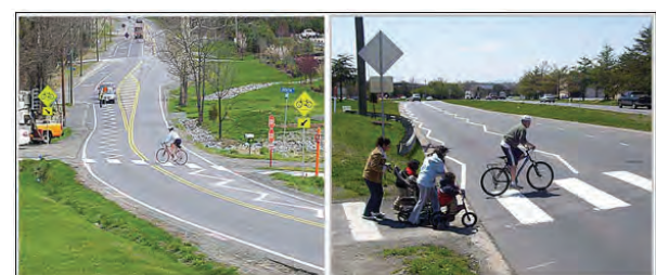
Zig-zag markings on Belmont Ridge Road (left) and Sterling Boulevard (right) in Loudoun County.
