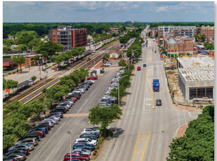
View of Northwest Highway, looking West
